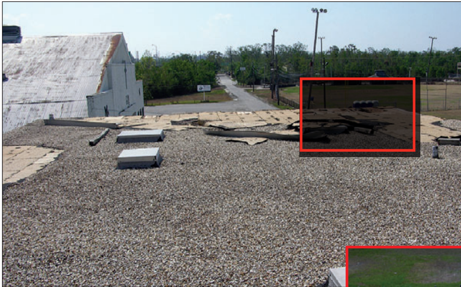
Figure 6-131: The built-up roof on this school was blown off after a few of the rotted wood planks detached from the joists. Estimated wind speed: 120 mph. Hurricane Katrina (Mississippi, 2005)
