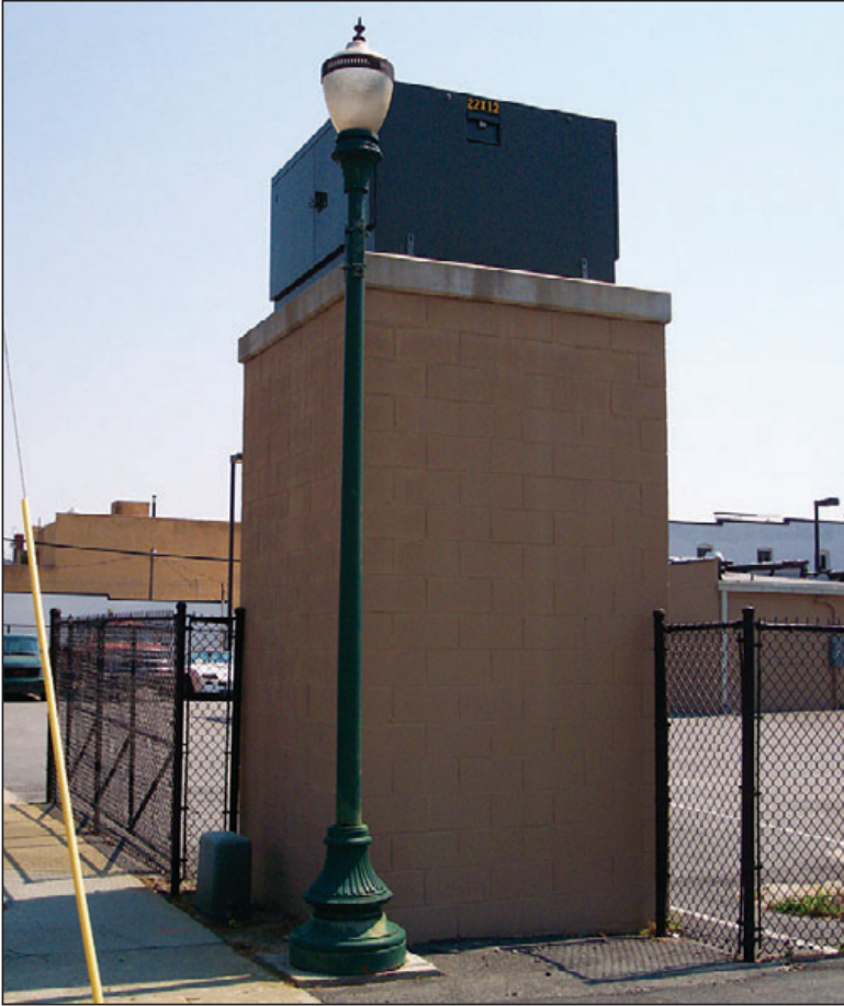
Figure 5-30: Utility component elevated above flood level
