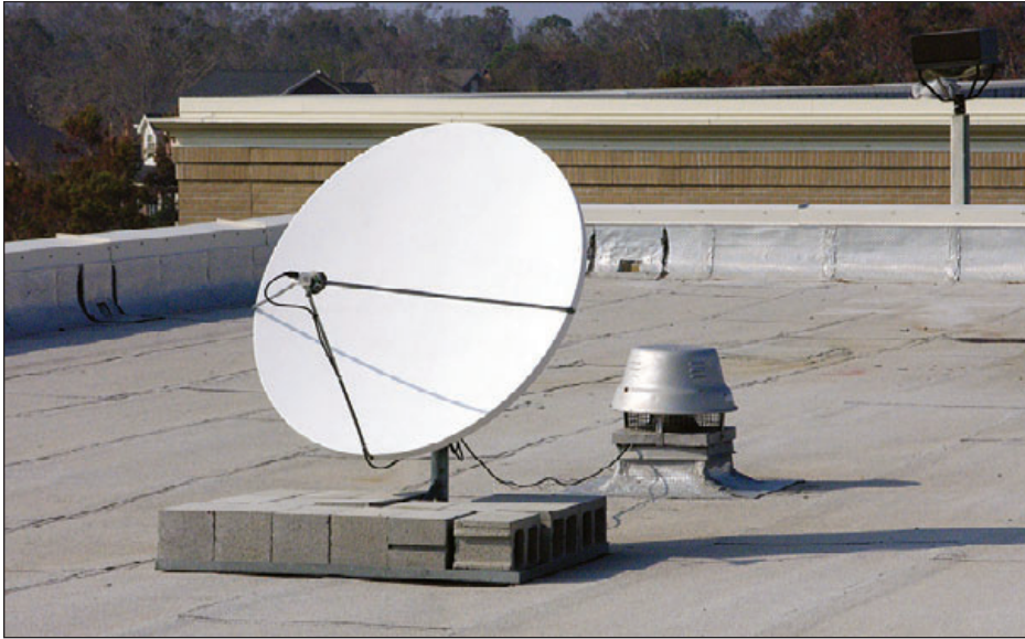
Figure 6-107: Common anchoring method for satellite dish. Estimated wind speed: 85–95 mph. Hurricane Ivan (Florida, 2004)
