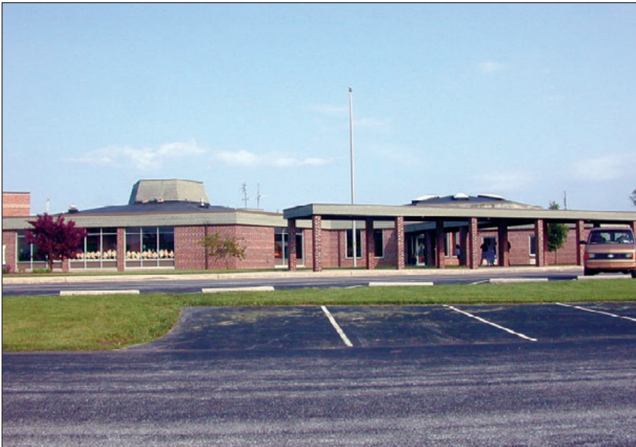
Figure 1-9: Elementary school, Fairfield, PA, 1980s
