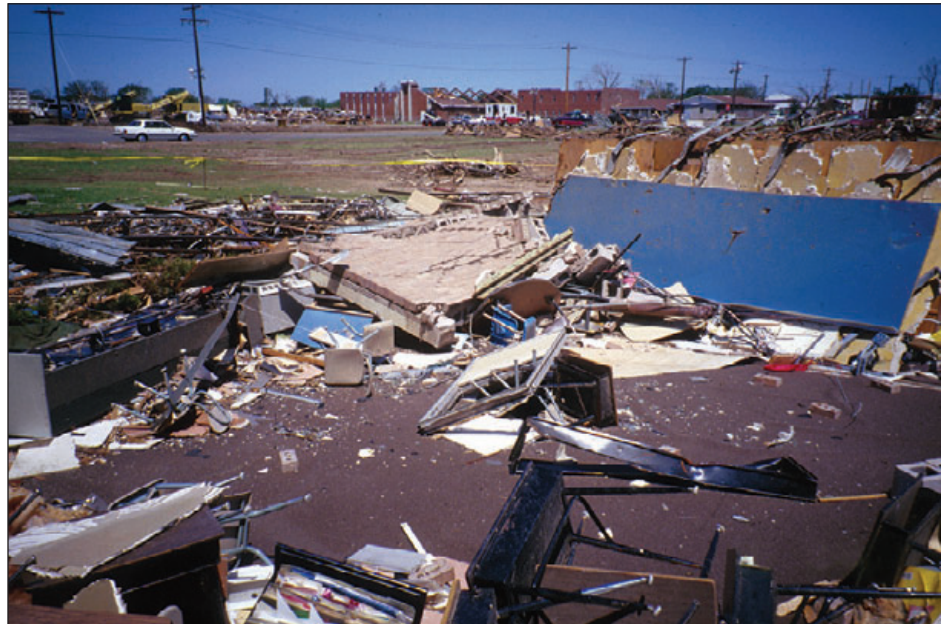
Figure 6-17: The roof and all of the walls of a wing of this elementary school were blown away by a violent tornado. (Oklahoma City, 1999)
