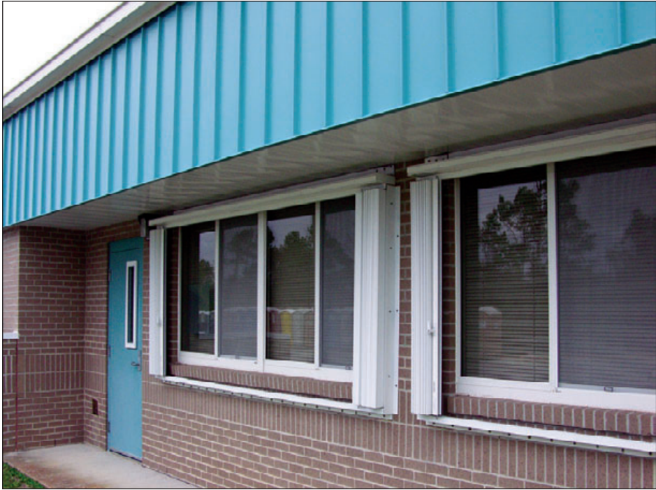
Figure 6-125: This school has accordion shutters. Estimated wind speed: 105–115 mph. Hurricane Ivan (Florida, 2004)
