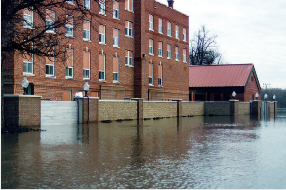
Figure 5-29: A masonry floodwall with multiple engineered openings in Fargo, ND, during flooding in 2001
