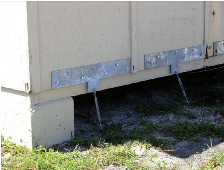
Figure 6-27: Unlike the portable classroom shown in Figure 6-22, with the thick T-shaped plates and taut turnbuckles, this portable classroom has a robust anchorage to the ground. Hurricane Francis (Florida, 2004)
