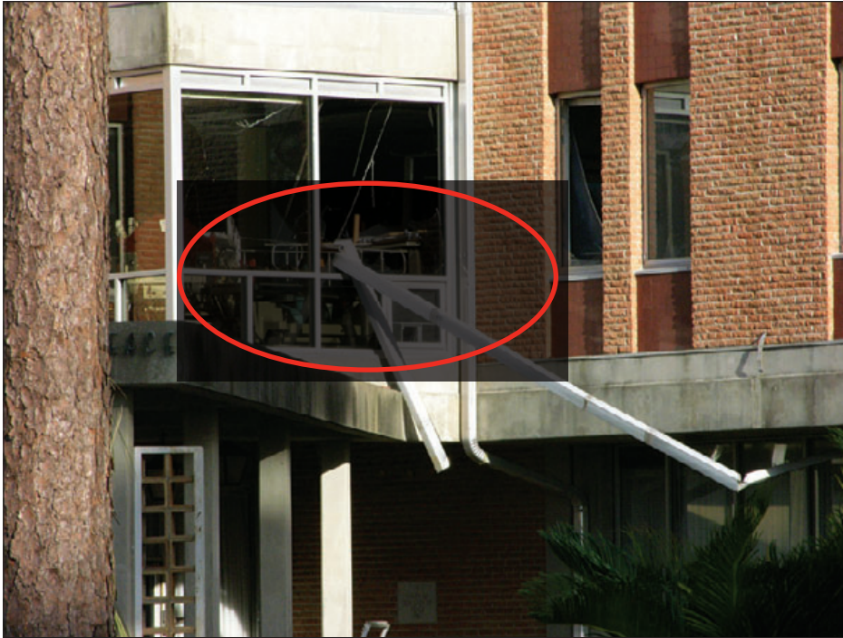
Figure 6-78: Blow-off of this downspout resulted in glazing breakage. Estimated wind speed: 105–115 mph. Hurricane Ivan (Florida, 2004)
