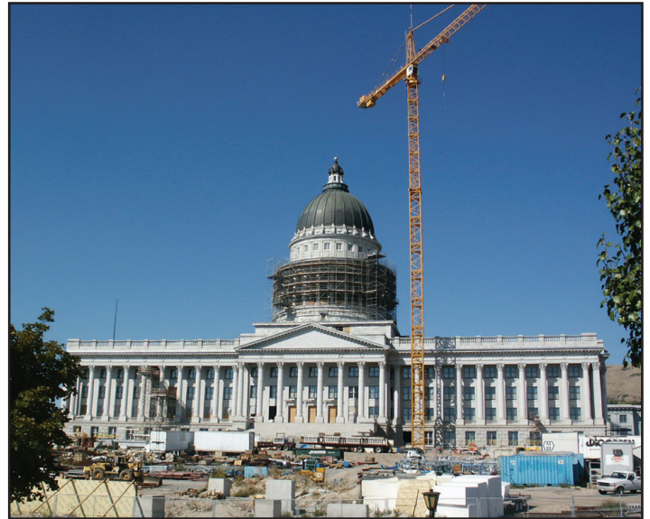
The State of Utah renovated the Capitol Building to preserve a historic building and to ensure public safety and continuity of government in the event of a large earthquake. The Capitol Building rests on a system of 265 seismic base isolators, separating the building from the foundation and lessening the effects of earthquake shaking. Photo taken September 24, 2006, courtesy of the Utah Geological Survey.
