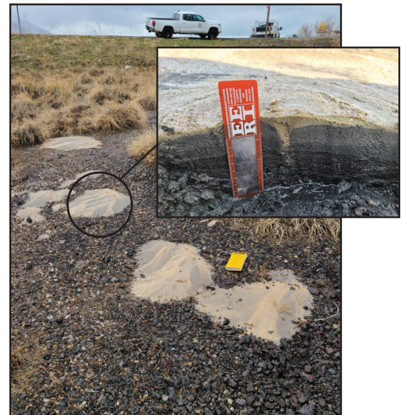
Sand boils near the Great Saltair event center caused by ground-shaking-induced liquefaction from the Magna earthquake. Photo courtesy of the Utah Geological Survey.
