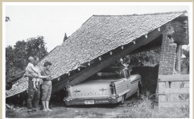
Ground shaking from the 1962 M 5.8 Richmond earthquake caused this brick garage to collapse onto a car. Photo courtesy of The Ogden Standard Examiner.
