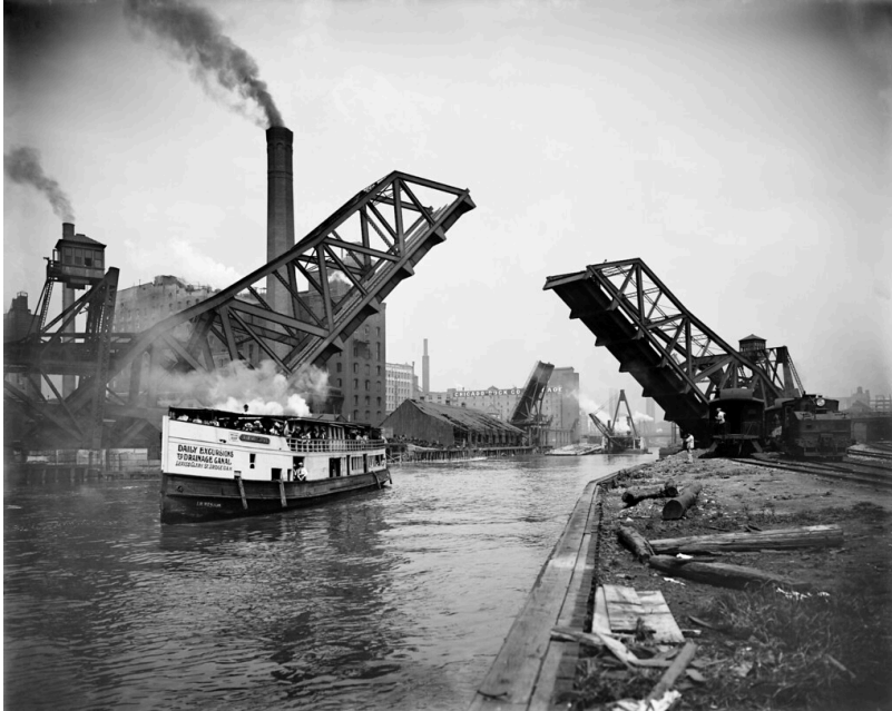
" 12th Street bascule bridge, Chicago, Illinois, ca. 1905 " by trialsanderrors is licensed under CC BY 2.0 .
